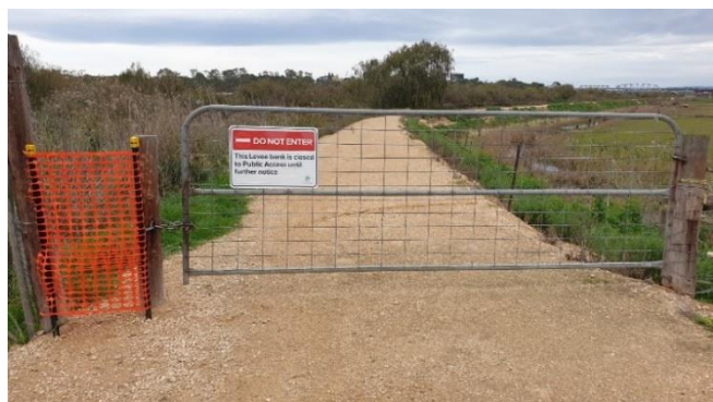
Photo: Restricted access to levee banks.
